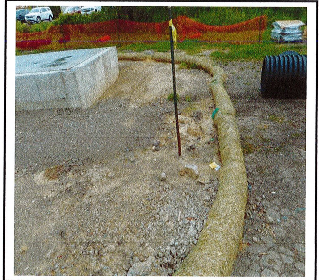
Sediment Barrier has been installed.
