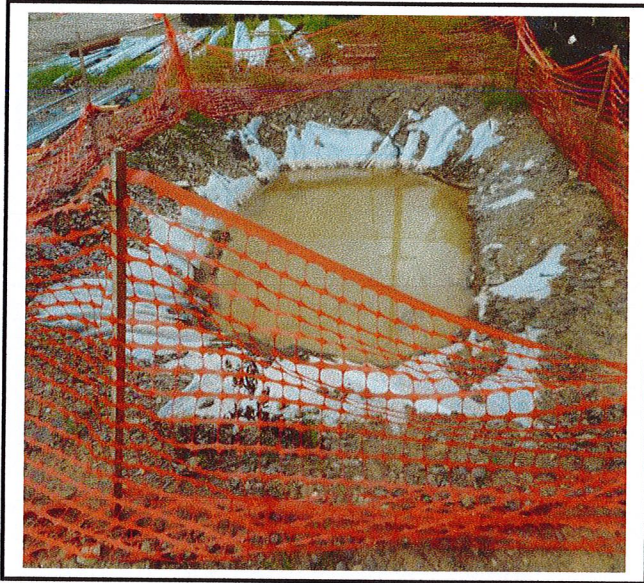
Concrete washout area.
