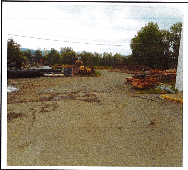
Construction entrance has been installed.
