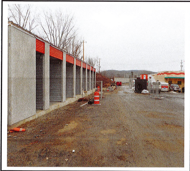
Monitor the amount of sediment being tracked out of the site.
