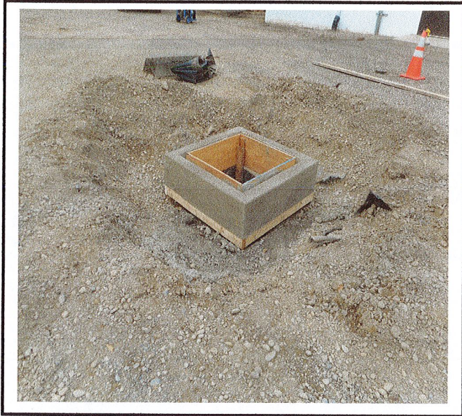
Drop inlet being brought up to grade.
