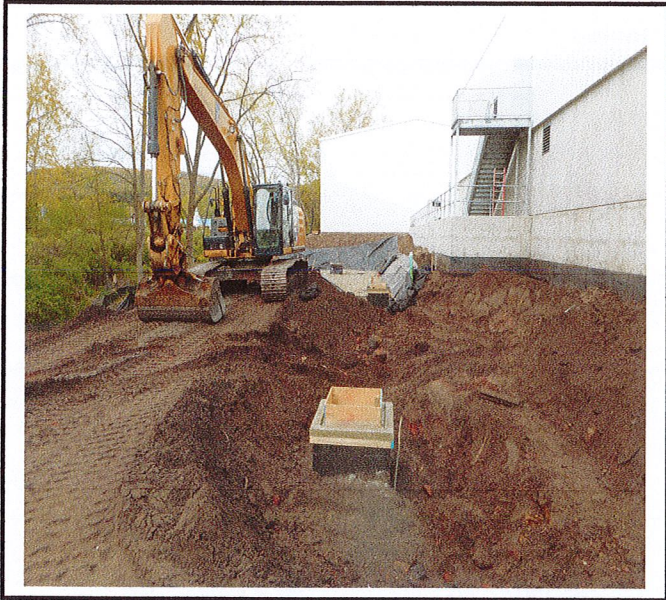
Bioretention under construction.
