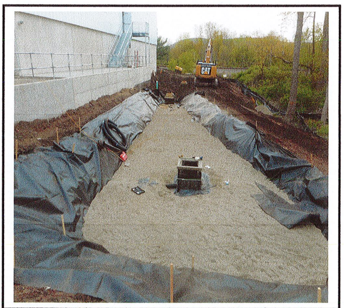
Bioretention on south end of property under construction
