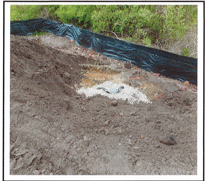
Outlet of bioretention on south end of property.
