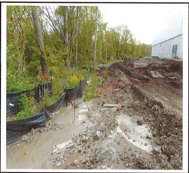
Silt fence functioning.
