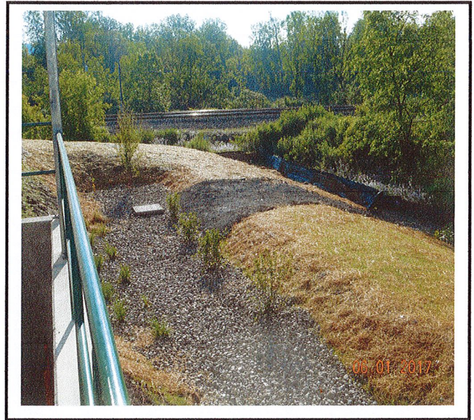
Finished bioretention #2 is complete.
