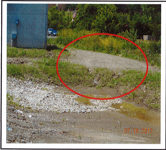
Erosion into unfinished stormwater basin.
